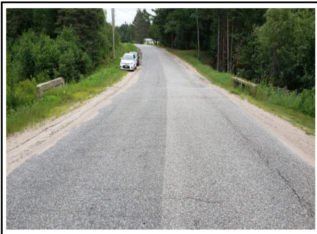
Photo 2 Structure from west approach
