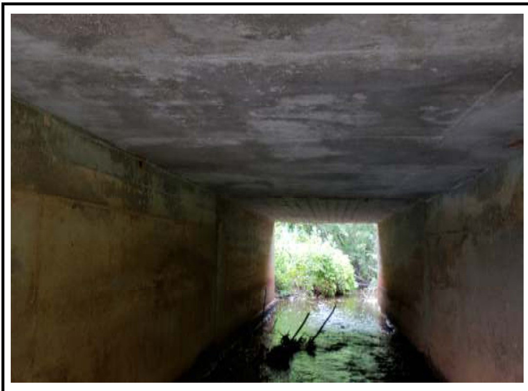
Photo 10 South underside of structure
