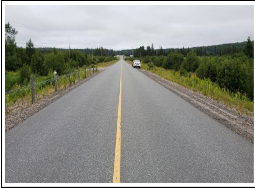
Photo 3 East approach from centre of structure
