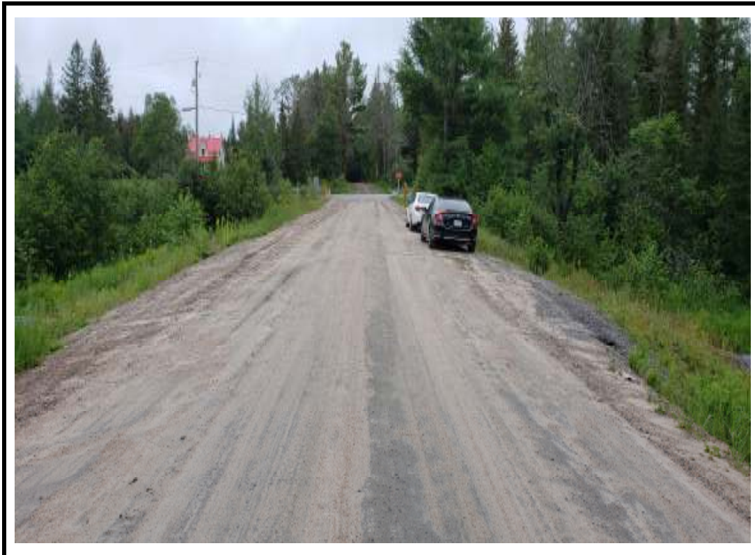
Photo 2 Structure from south approach
