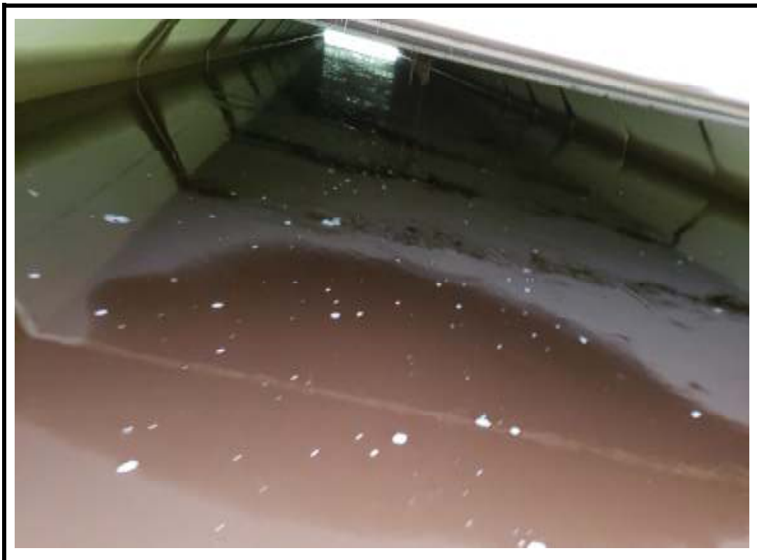
Photo 10 Visible portion of interior barrel
