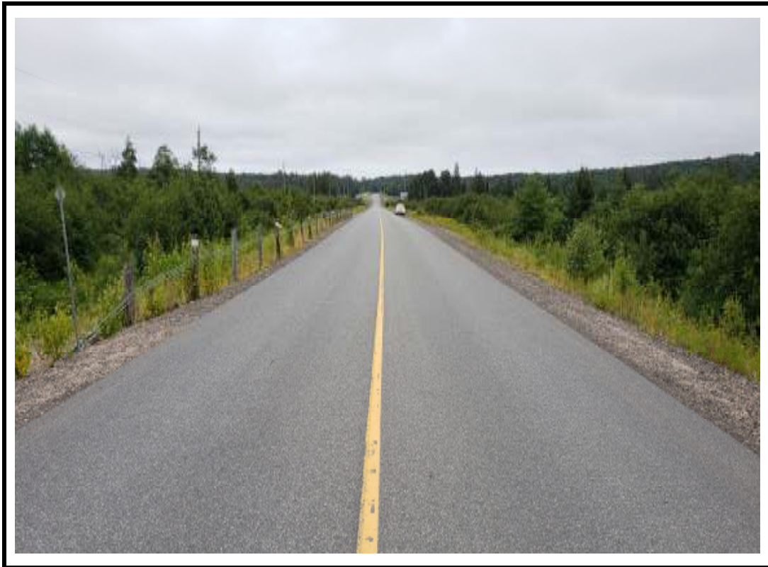
Photo 2 Structure from west approach
