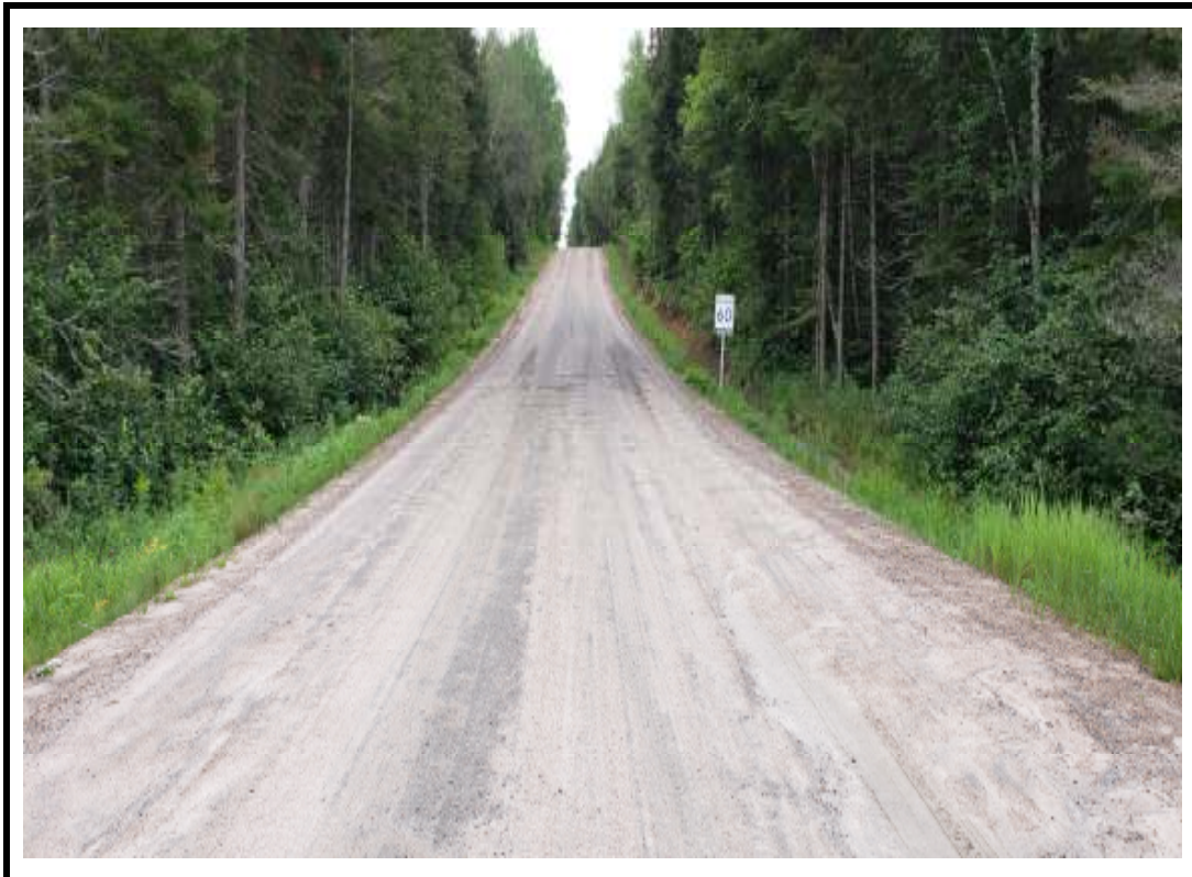
Photo 4 South approach from centre of structure
