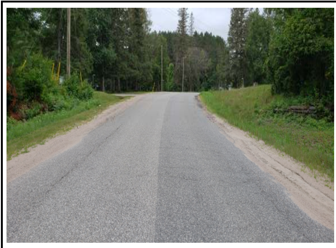
Photo 4 West approach from centre of structure
