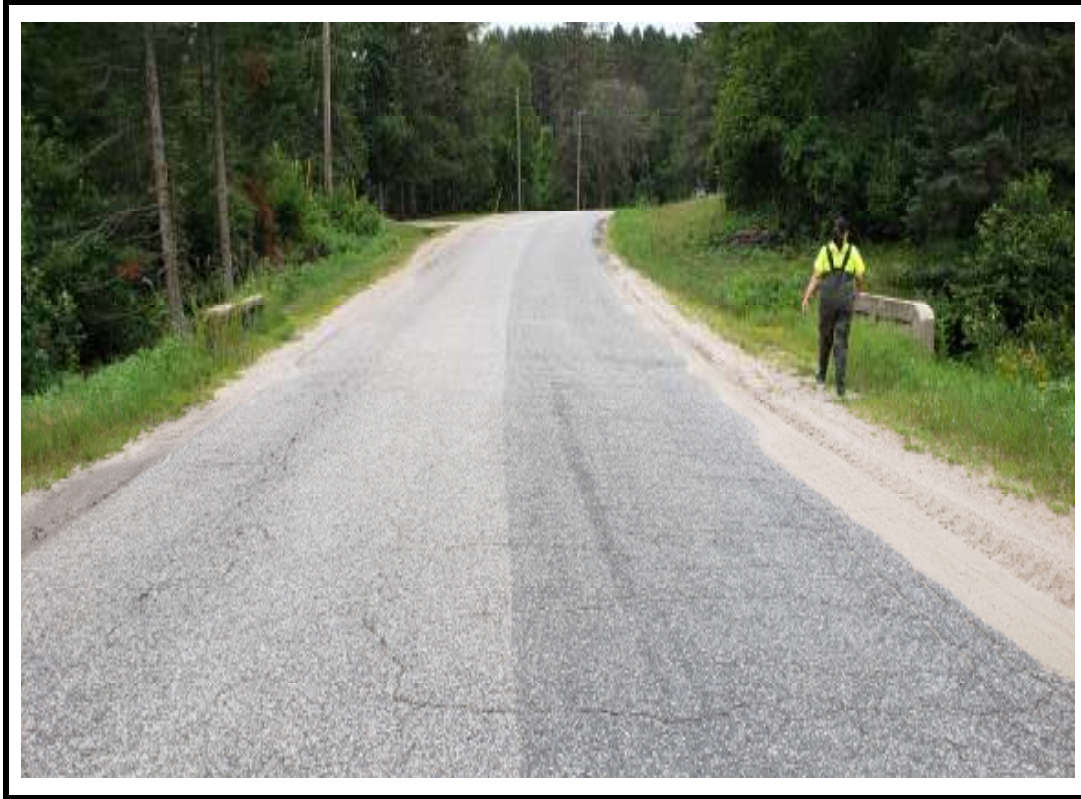
Photo 1 Structure from east approach
