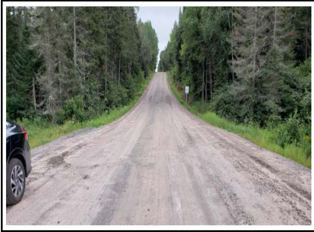
Photo 1 Structure from north approach
