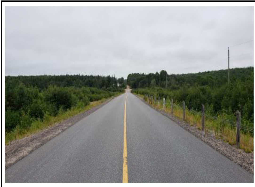
Photo 4 West approach from centre of structure
