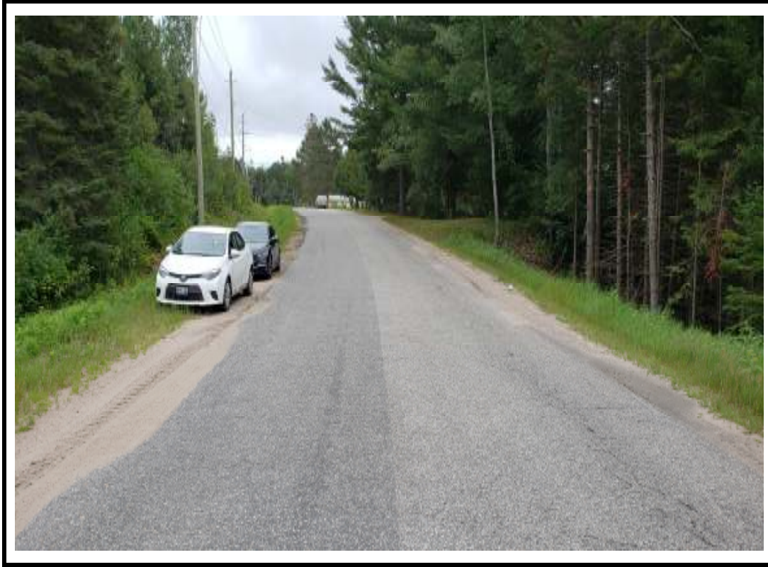
Photo 3 East approach from centre of structure
