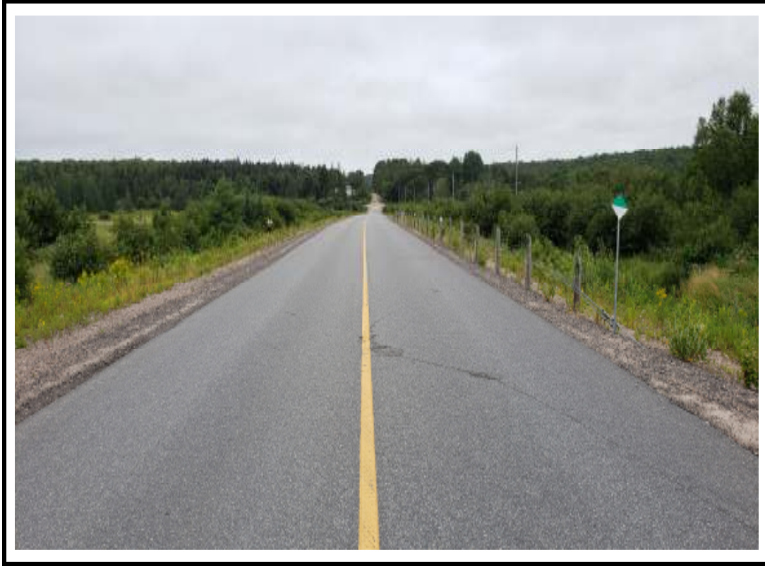
Photo 1 Structure from east approach
